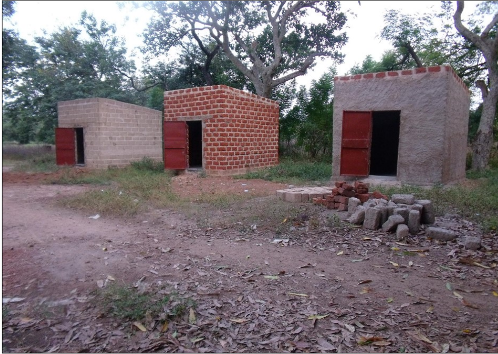
Figure 1. The concrete stone house, the red-stone house and the mud-house dimension 2.5 x 3 m in ground area.
